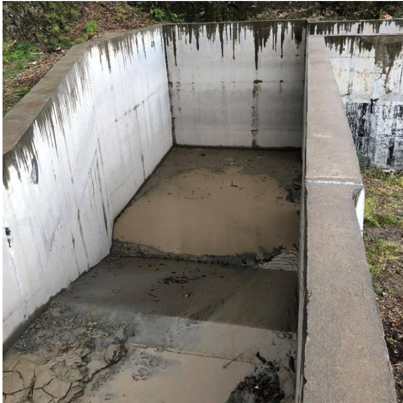
Siphon Inlet Pond
