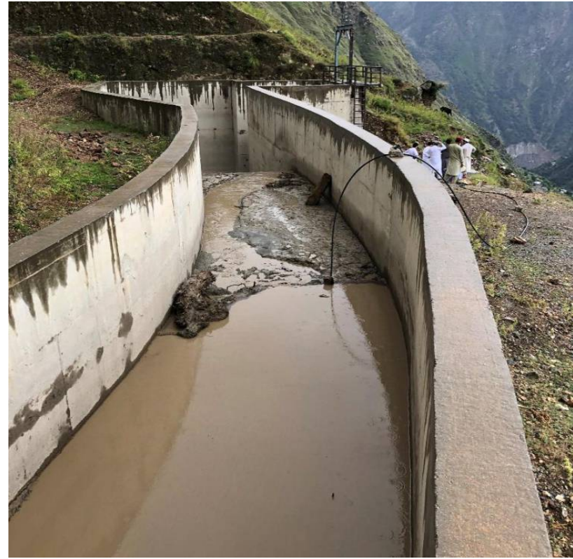
Siphon Inlet Pond
