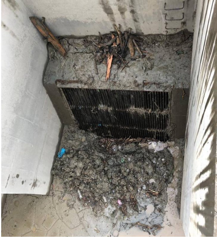
Siphon Inlet Pond
