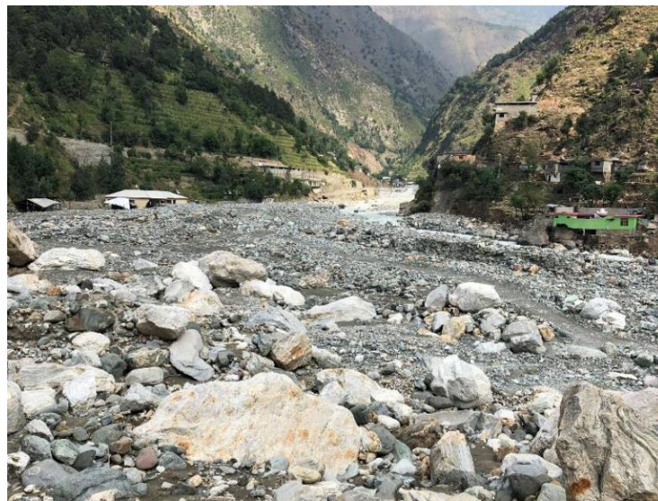
Access Road u/s Powerhouse
