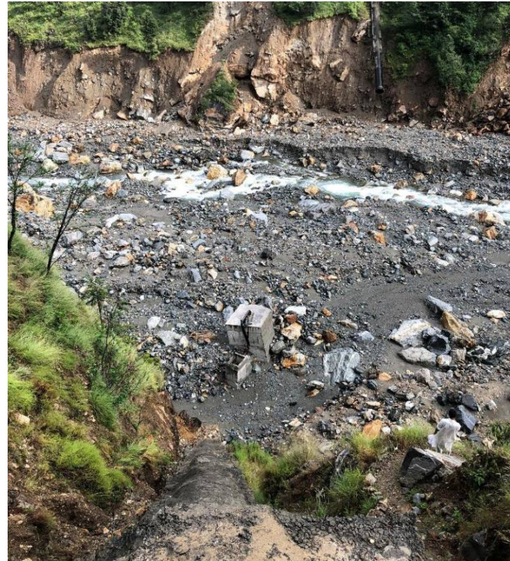
Siphon Drainage Valve
