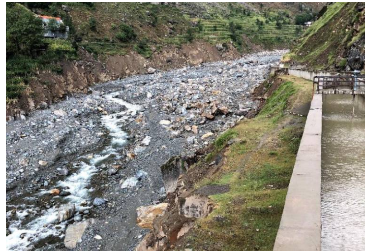
Weir Access Road near Gravel Trap
